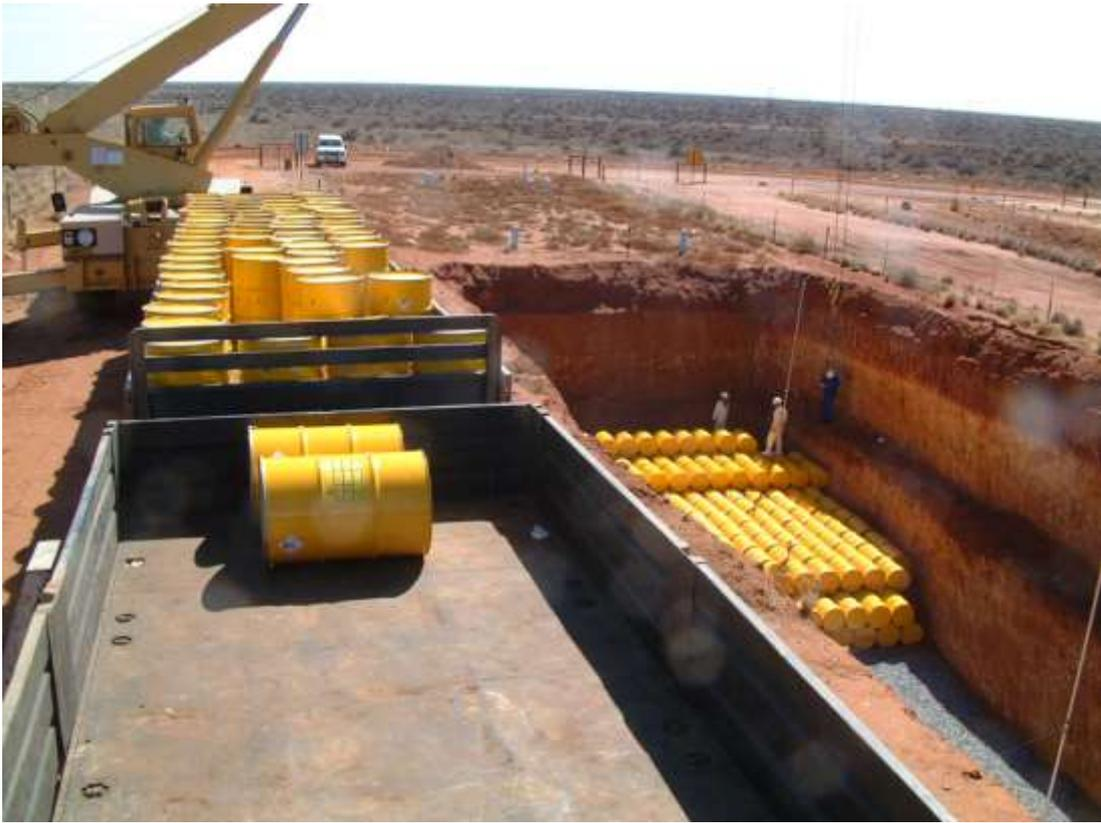
**Figure 5: Disposal of waste packages into near surface trenches**
