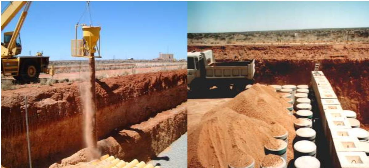
**Figure 6: Backfilling of near surface trenches after emplacement of waste packages**
