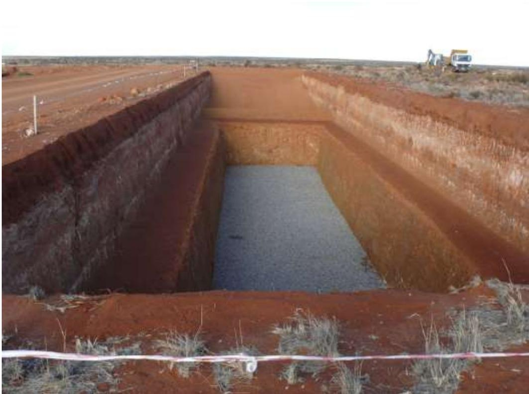
**Figure 2: LLW near-surface disposal trench at Vaalputs**
